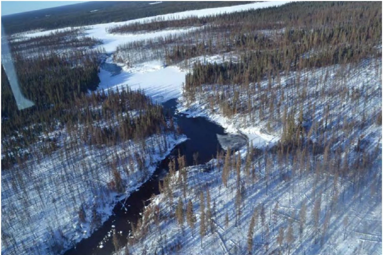
Figure C: View of Birch River Crossing Location (Looking North)
