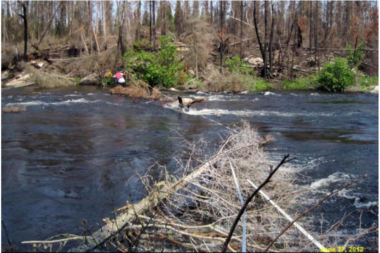
Figure D: View of Birch River Crossing – North Abutment
