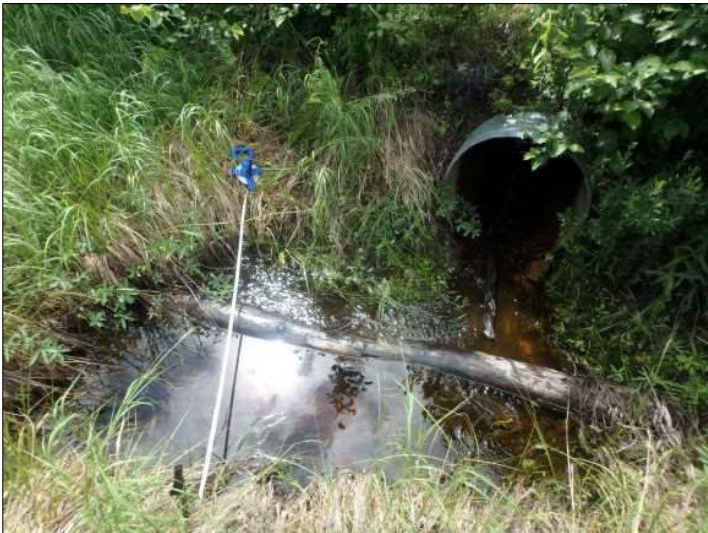
Culvert inflow (Jul. 20, 2019)
