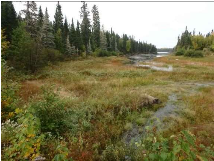
Facing downstream at culvert (Sep. 17, 2019)
