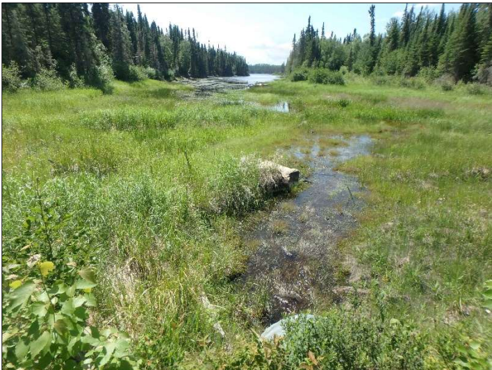
Facing downstream at culvert (Jul. 16, 2019)
