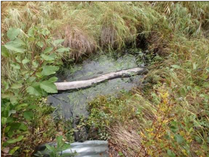
Culvert inflow (Sep. 17, 2019)
