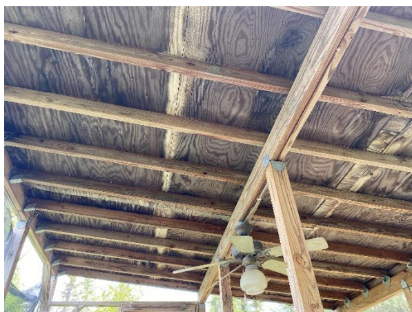
Plate 24: Roof Supports of Enclosed Front Porch
