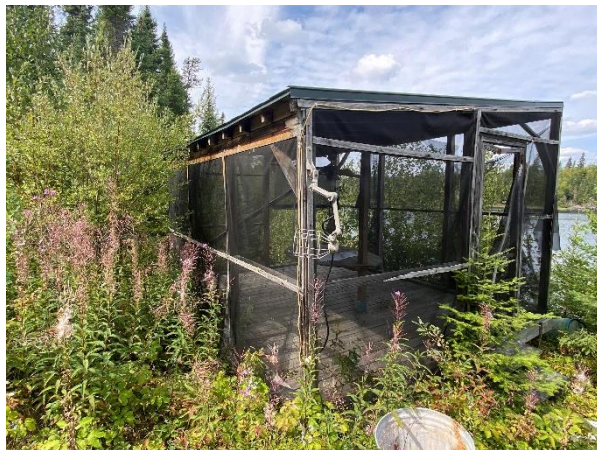
Plate 22: Enclosed Front Porch
