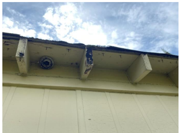
Plate 14: Protruding Rafters
