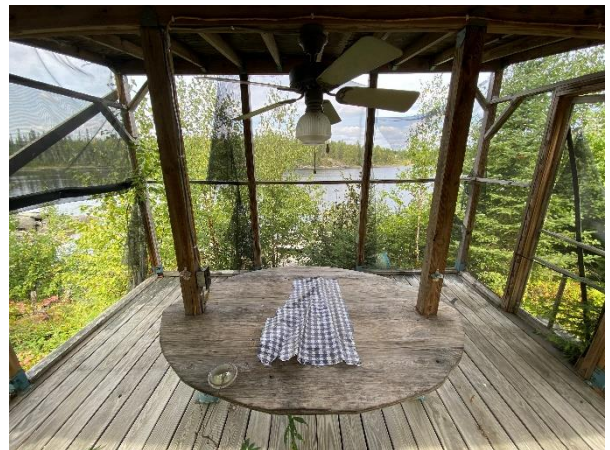
Plate 23: Interior of Enclosed Front Porch
