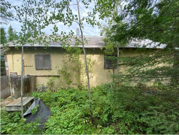
Plate 9: North Elevation of the Cabin
