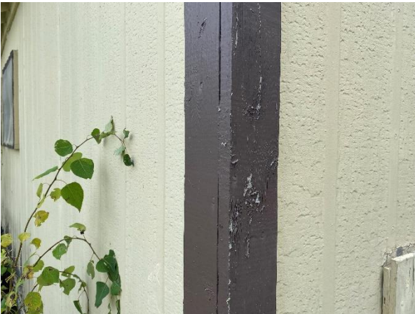
Plate 11: Timber Corner Post
