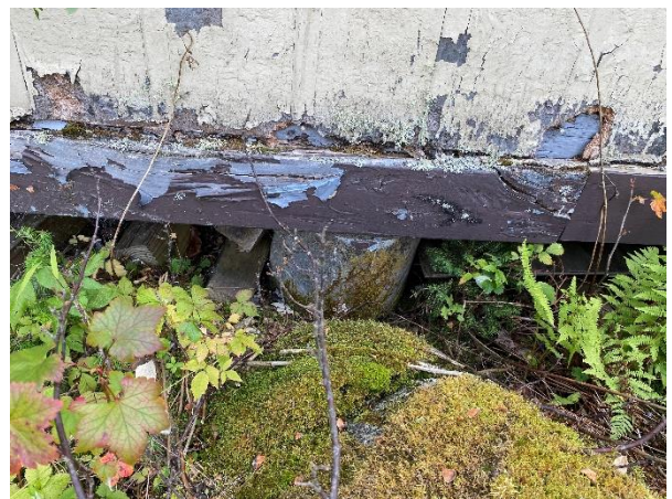
Plate 20: Concrete Foundational Supports
