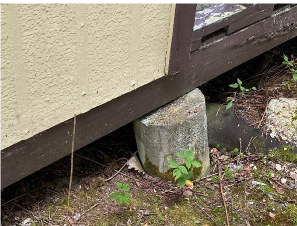
Plate 19: Concrete Foundational Supports
