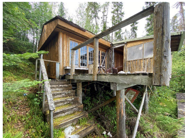
Plate 4-6: Oblique View of Hunting Cabin
