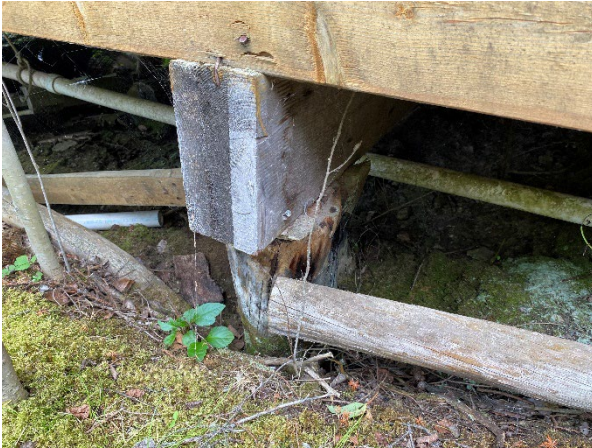
Plate 4-13: Cabin Floor Joists
