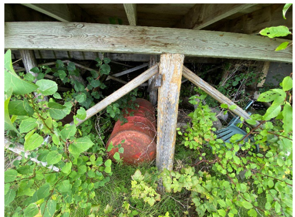
Plate 4-12: Dimensional Lumber and Wood Beam Cabin Supports
