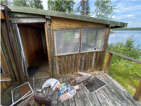
Plate 4-7: Cabin Porch and Entranceway
