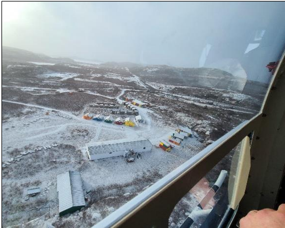
Figure 12-1: Aerial view of Hope Brook camp
